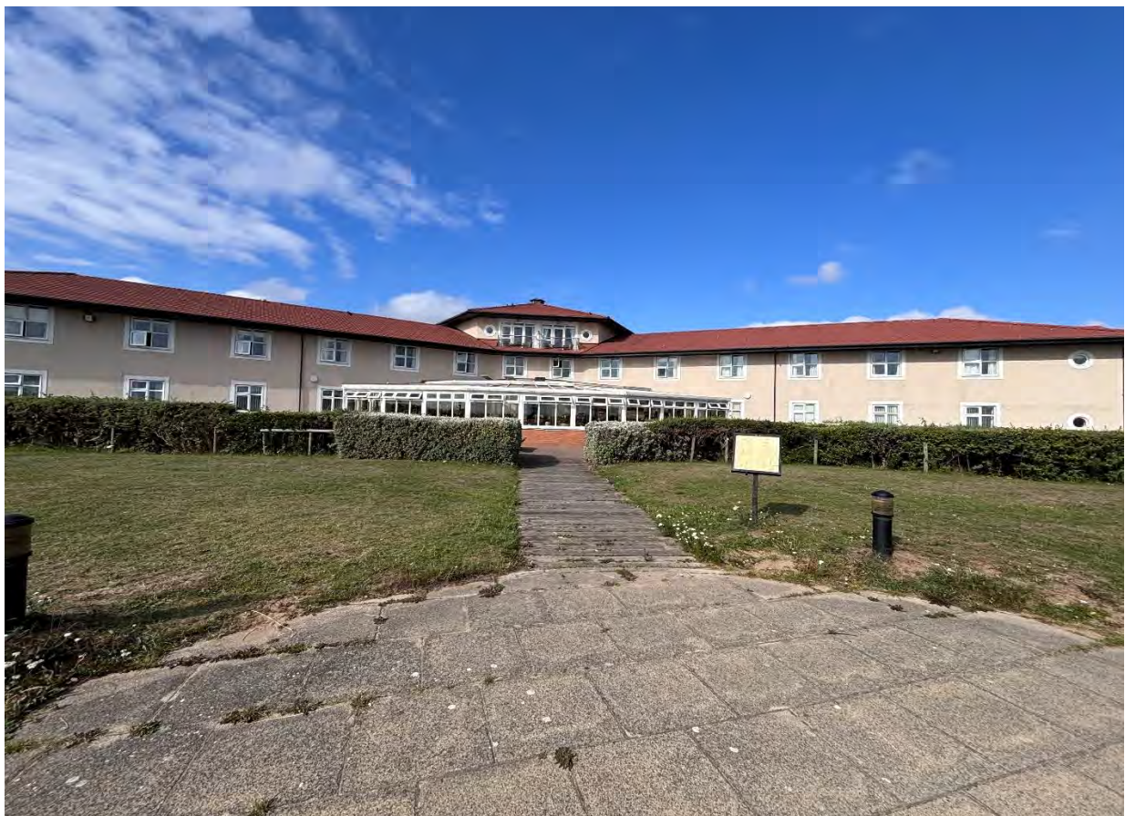
Photo 12 Eastern elevation of Site
