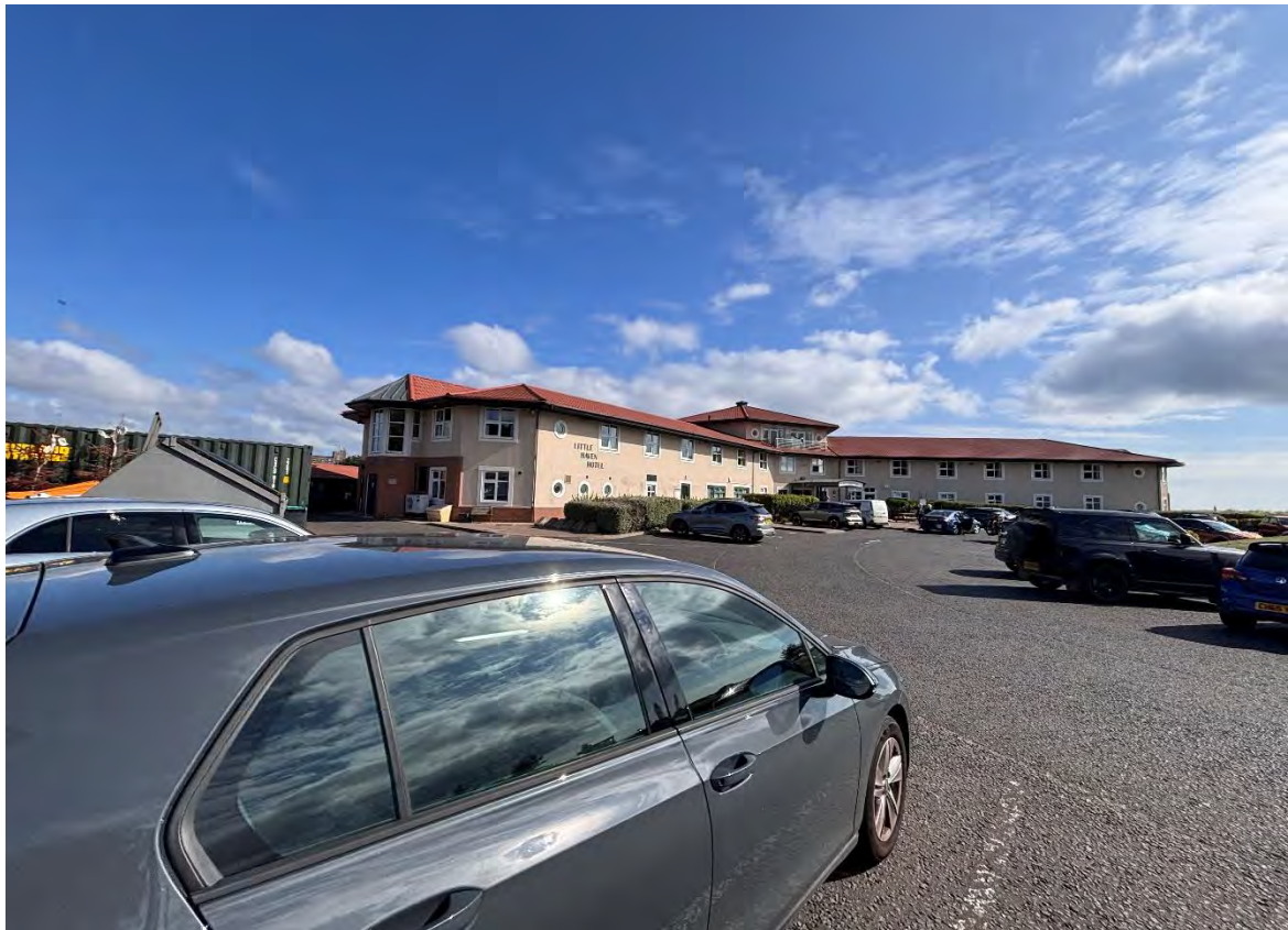
Photo 6 Looking northeast from southwest of Site showing hotel southern elevation
